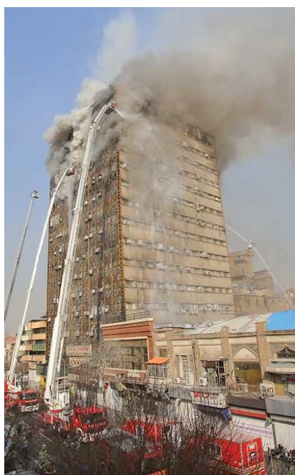
Fig. 2. The 17-story Plasco Building in Tehran which was engulfed by a fire and fully collapsed on January 19, 2017
